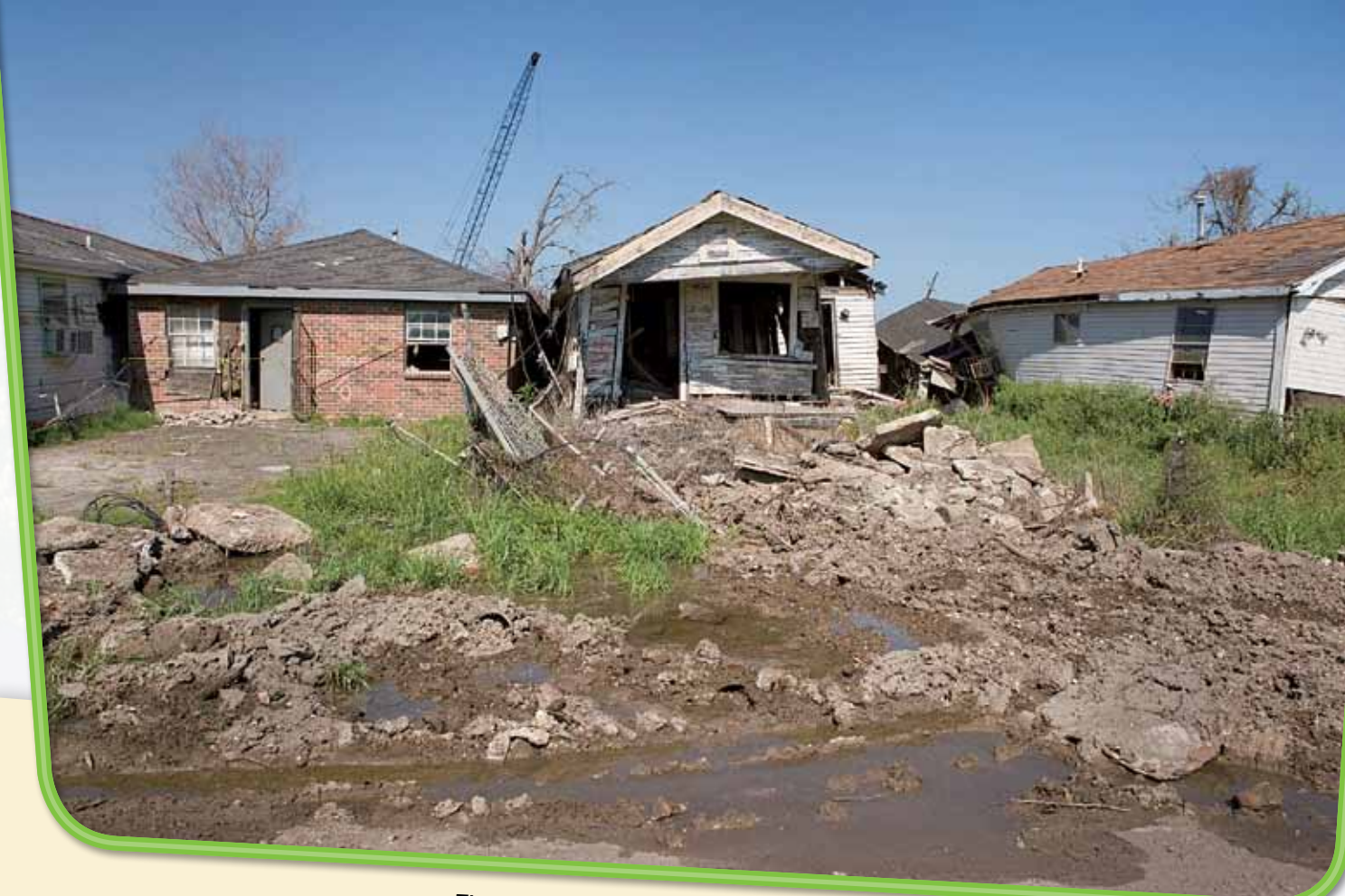
These homes in New Orleans collapsed during flooding from the storm surge caused by the high winds of Hurricane Katrina.
